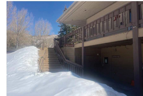
The pavilion has two stories that can be accessed from the outside. A tiered staircase connects the two levels.
