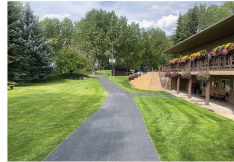
There is an asphalt walkway from the Pavilion Park parking lot that runs past the pavilion and turns into a crushed granite path.
